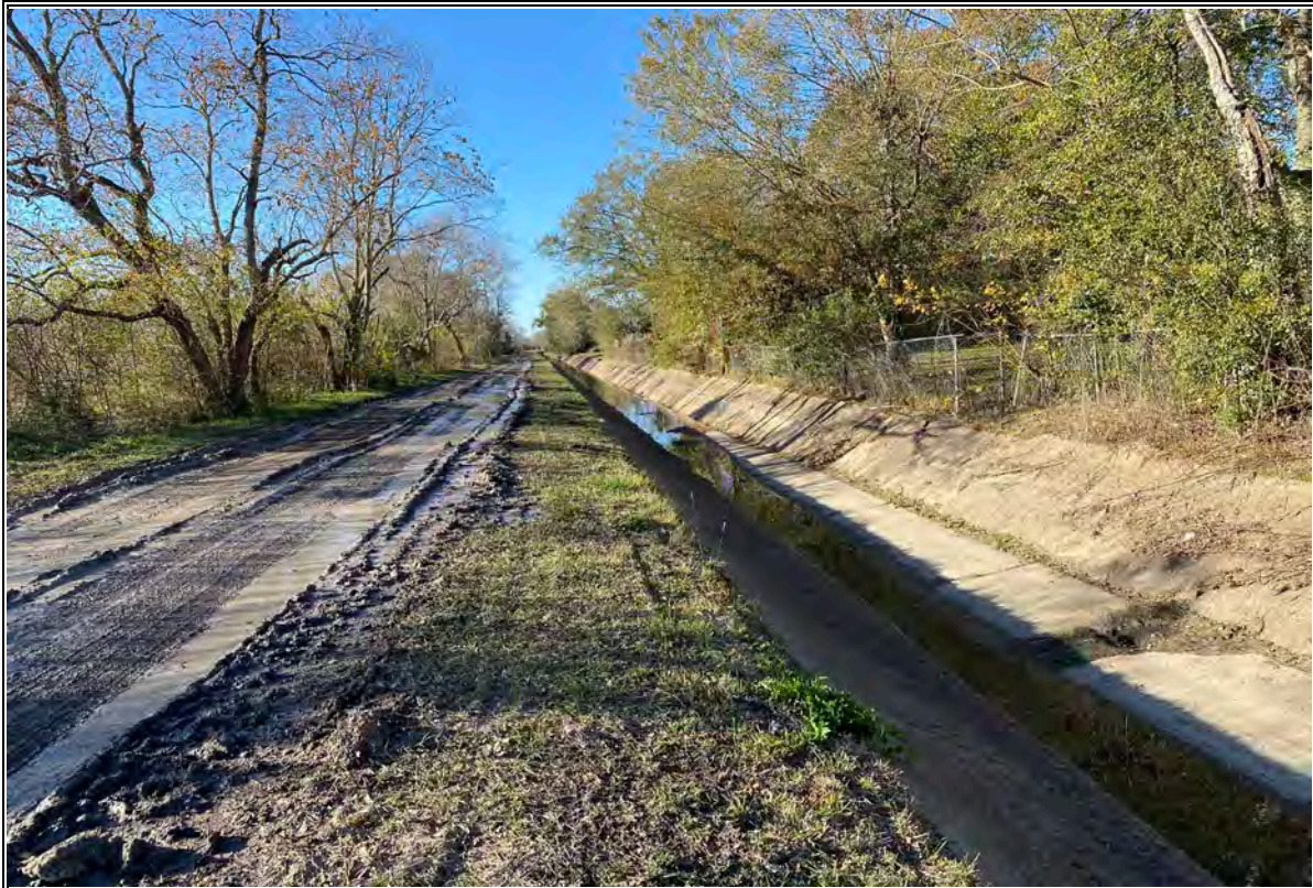
View of eastern boundary of subject property and JCDD7's A3A drainage ditch, facing north.
